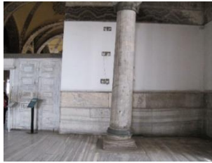
(b) Inclination of column
