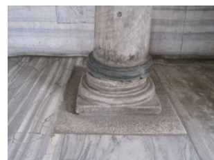
(c) Sliding of the column
